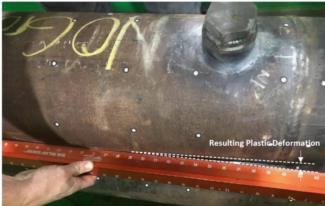
Figure 4-4: Photograph showing resulting plastic deformation of the temporary repair.
