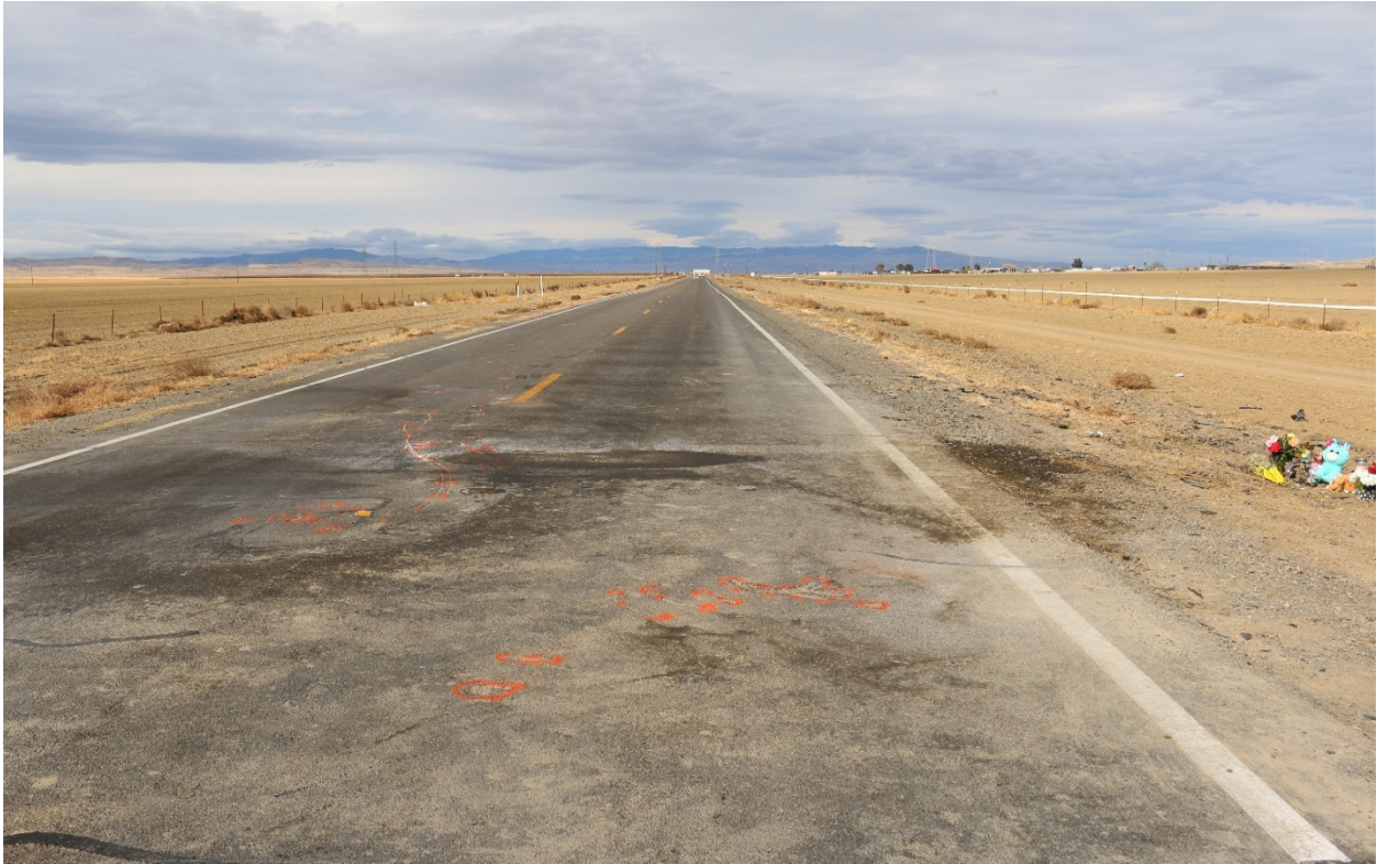
Figure 5: Northbound view of SR-33 depicting tire marks, fluid debris, scrapes, and gouges in the northbound lane. (Source: California Highway Patrol).
