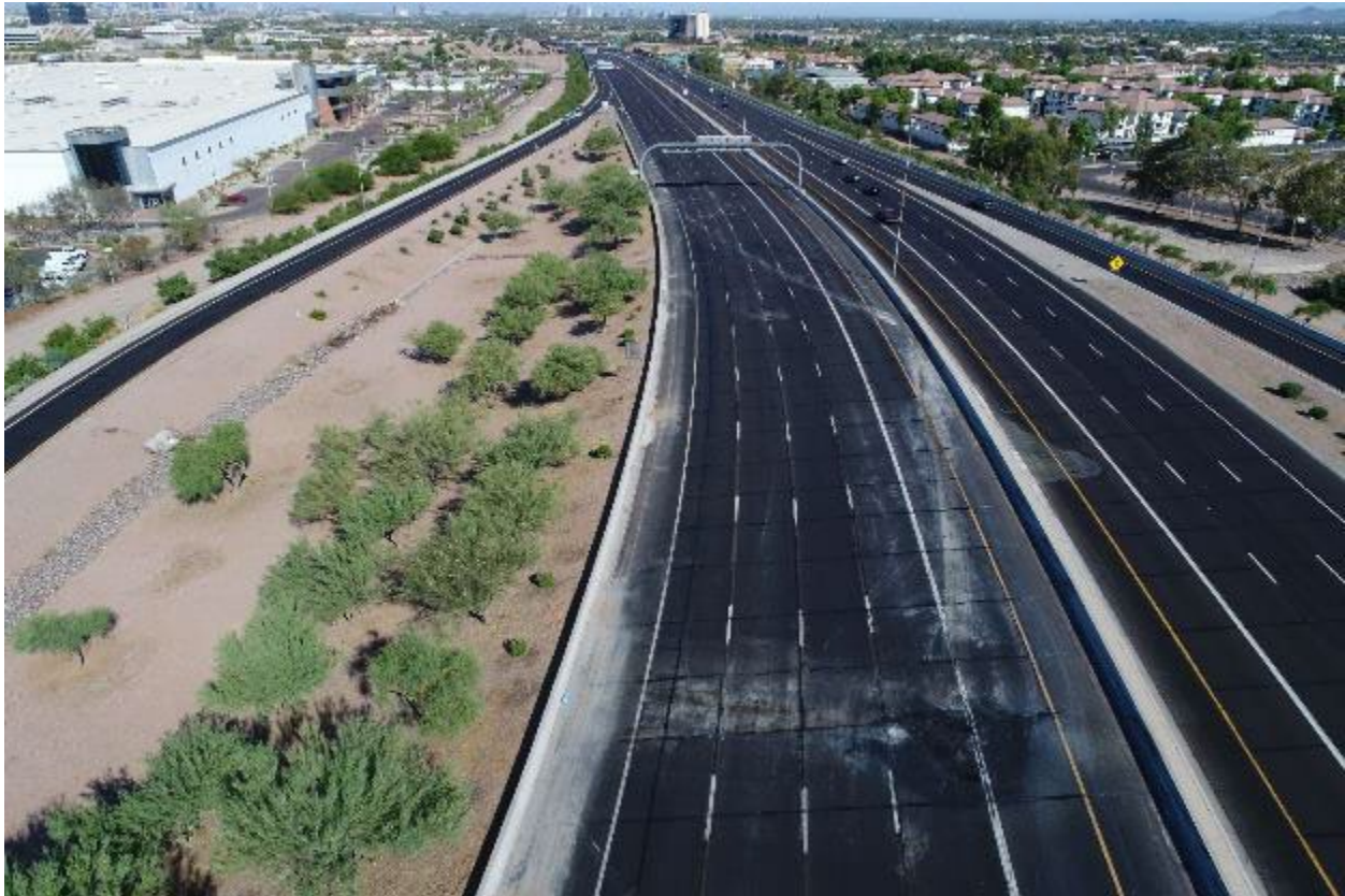
Figure 4: Aerial image of the eastbound travel lanes of SR-202 looking westbound.
