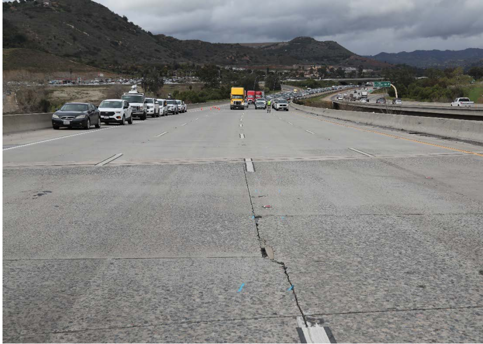
Photo #3 On-scene traffic control performed by CHP (Source CHP)
