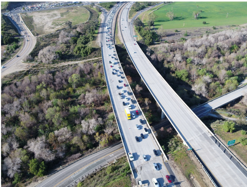
Photo #4 Overhead view of traffic control performed by Caltrans (Source: CHP)
