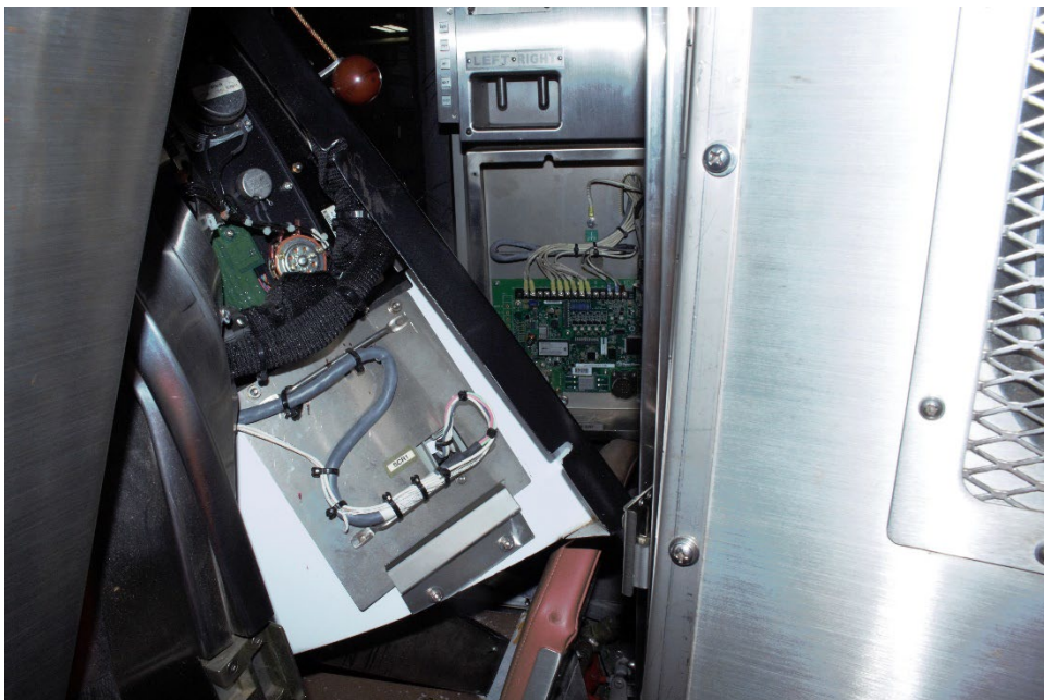
Photo 8 A close-up of the interior of lead train car showing the damage to the operator's cab and the loss of survival space due to the collision with the snow removal vehicle. (Source: NTSB)
