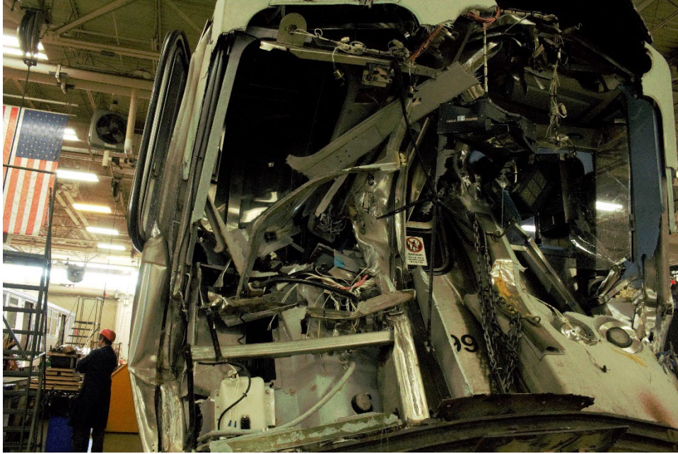
Photo 7 Photograph showing a close-up of the exterior damage to the lead train car and the loss of survival space caused by the extensive intrusion into the space resulting from the collision with the snow removal vehicle. (Source: NTSB)
