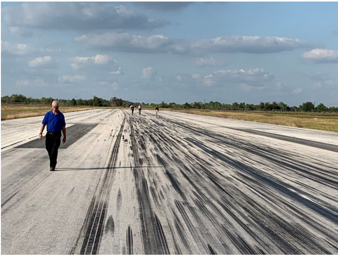
Figure 2. View down Runway 36 towards airport perimeter fence
