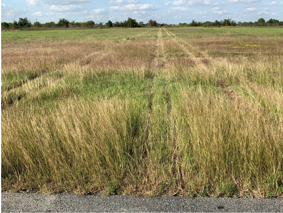
Figure 3. View past Runway 36 towards airport perimeter fence
