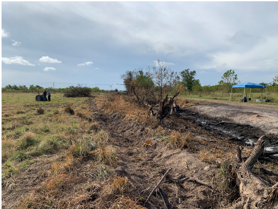
Figure 8. View looking back towards Morton Road
