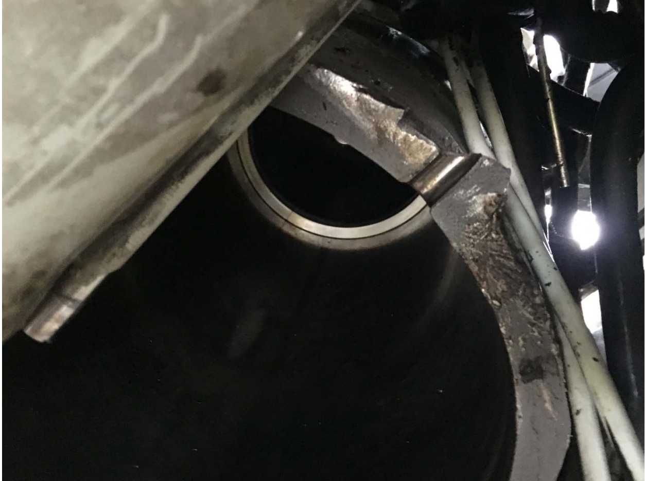
Figure 9 – Fracture surface on the lower section of the left main landing gear cylinder exhibiting features consistent with fatigue
