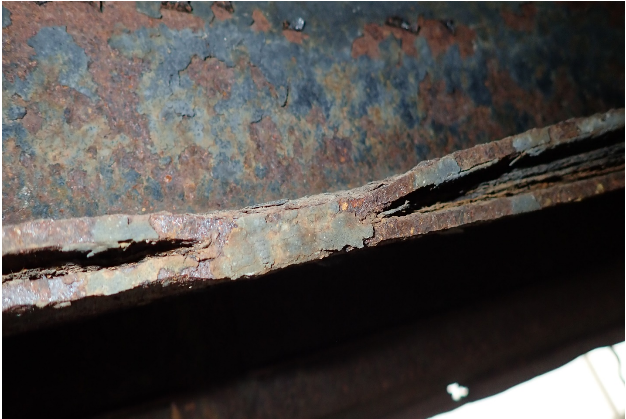
Vehicle Photograph: 3 - 2001 Ford Excursion Limousine – Image shows a spot weld joining the two frame rails.
