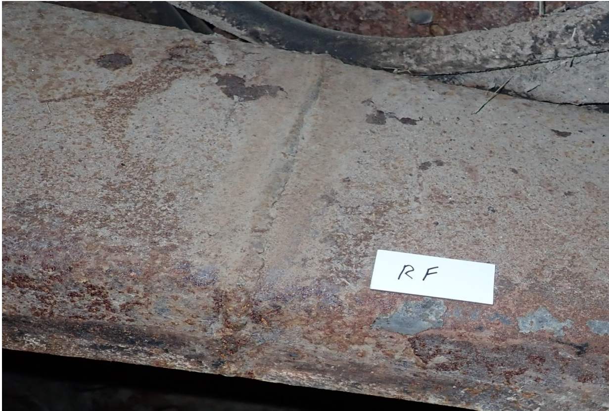
Vehicle Photograph: 5 - 2001 Ford Excursion Limousine – Image shows the weld joining the extension frame rail to the original frame rail at the right front of the vehicle.
