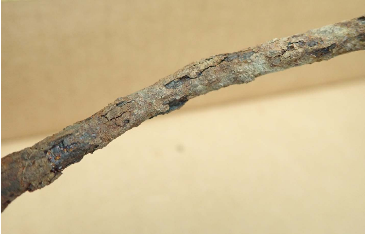
Figure 27: Corroded Steel Tubing Removed from Rear Brakes of Limousine
