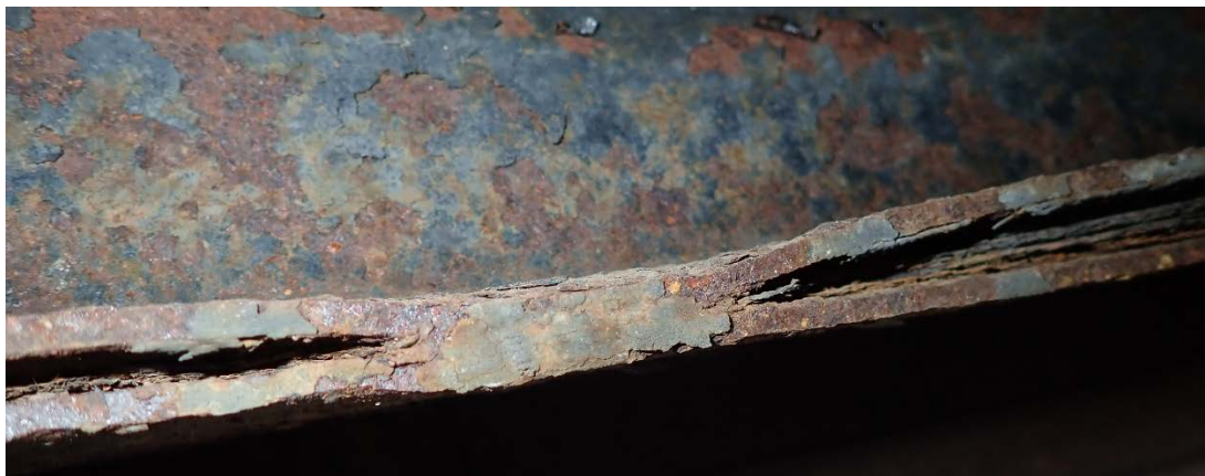
Figure 4: Spot Weld Joining Two Rails
