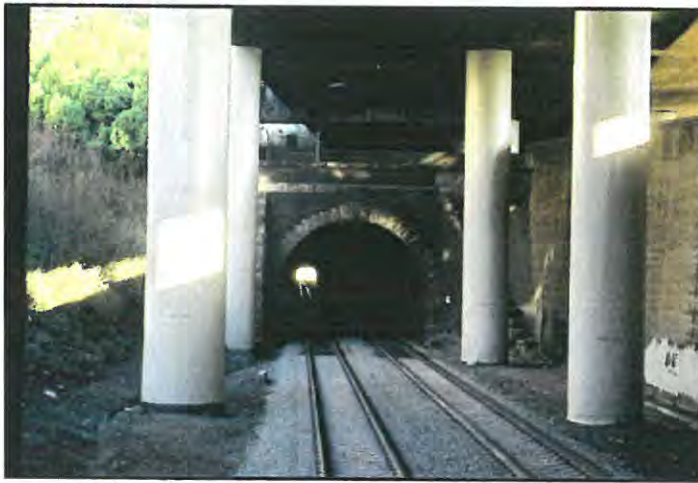
Figure 15: Tunnel south of San Francisco, FCA photo
