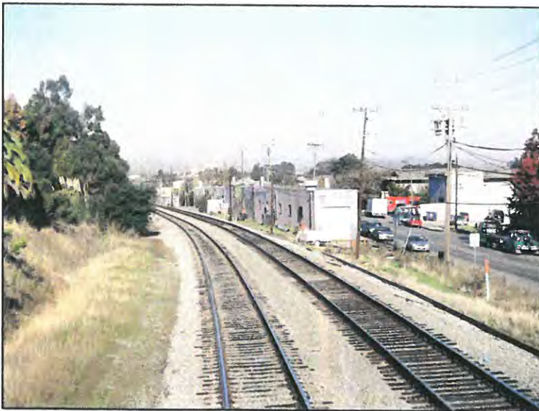
Figure 2: Typical Caltrain ROW through San Mateo County, FCA photo
