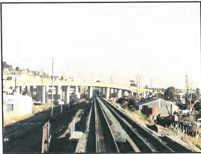
Figure 22: Bridge over Caltrain tracks, FCA photo
