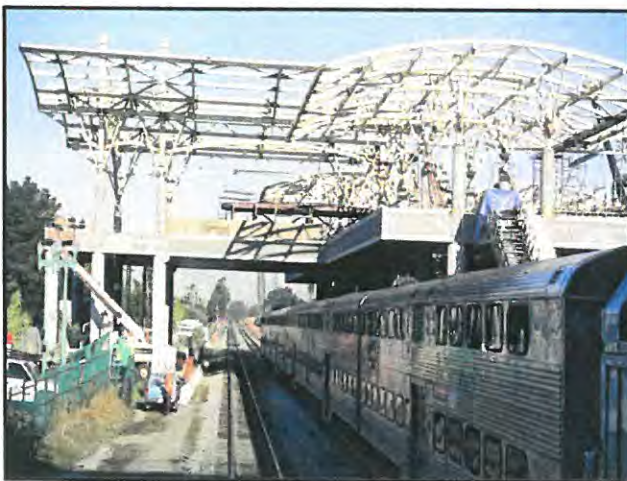
Figure 11: Bi-modal cat at BART station under construction, FCA photo
