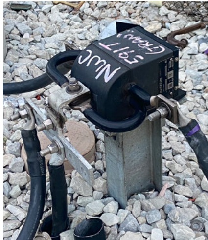
Figure 1: Signal Bond
