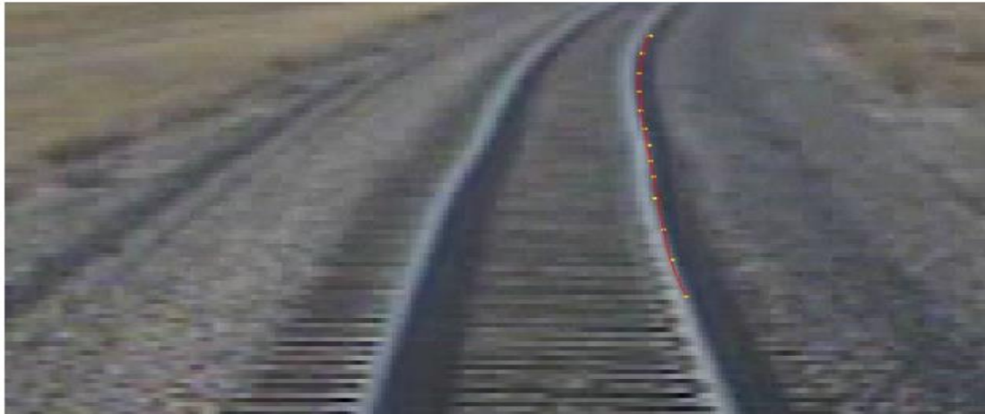
Image #2 from Amtrak Train No. 7 depicting track deviation. The lack of resolution is evident.
