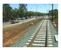
F.  $\underline{\text{Spur}} - \text{A}$  secondary track with access from only one end.
