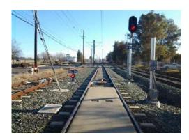
P. <u>Traffic Indicator Signal</u> – A fixed signal that displays a yellow "T" to indicate when traffic signals permitting LRV movement are displayed. Traffic controls prohibiting turns that conflict with LRV movement are not displayed.
