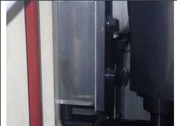
Guide shoe inspection
