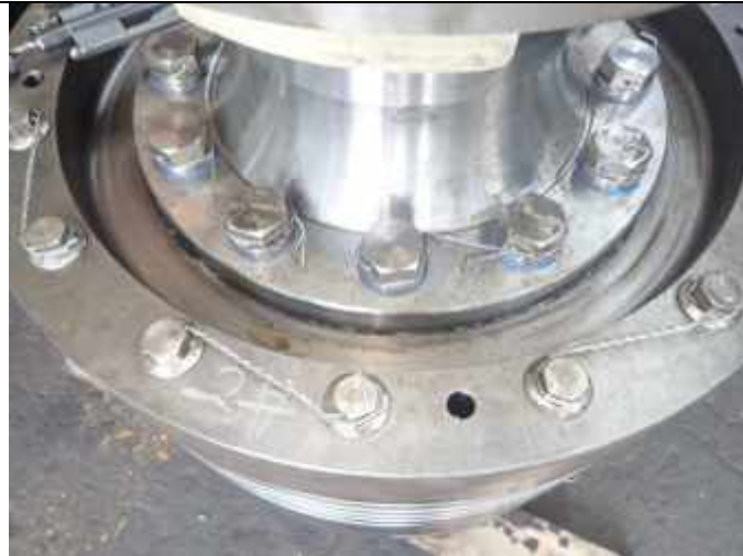
Penetration test of roller guide
