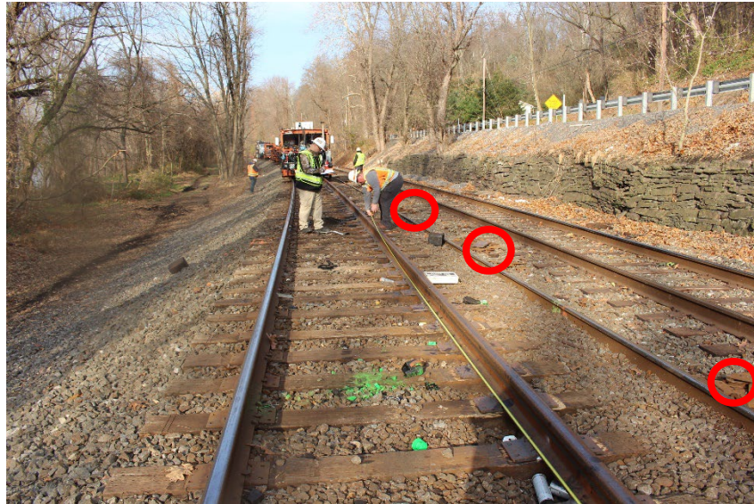
Figure 7 Photograph, looking north, of the track environment to include debris piles (circled in red) lying on the east side of the track and the sloping descent of the terrain on the west side of the track. (Source: NTSB)
