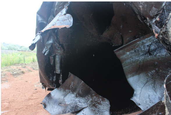
5(c) A-end breached area.
