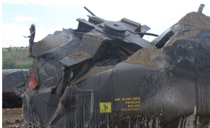
1(b) A-end, bottom buckled at inboard end of the stub sill.
