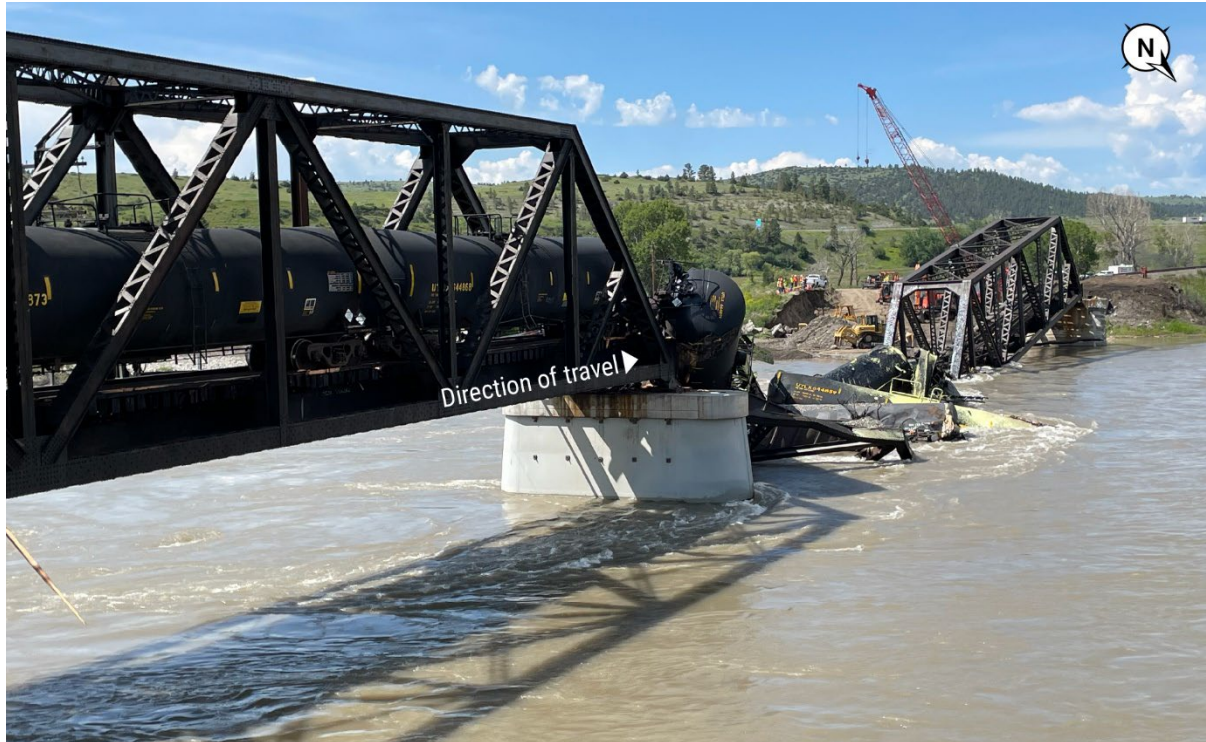
Figure. View of the accident scene.
