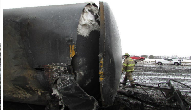
4 (b) A-end left side showing head shield separation and impact damage.
