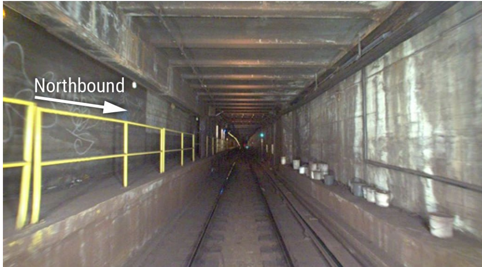
Figure 1. Photograph of the tunnel looking northbound toward the accident location and the 34th Street-Herald Square Station.
