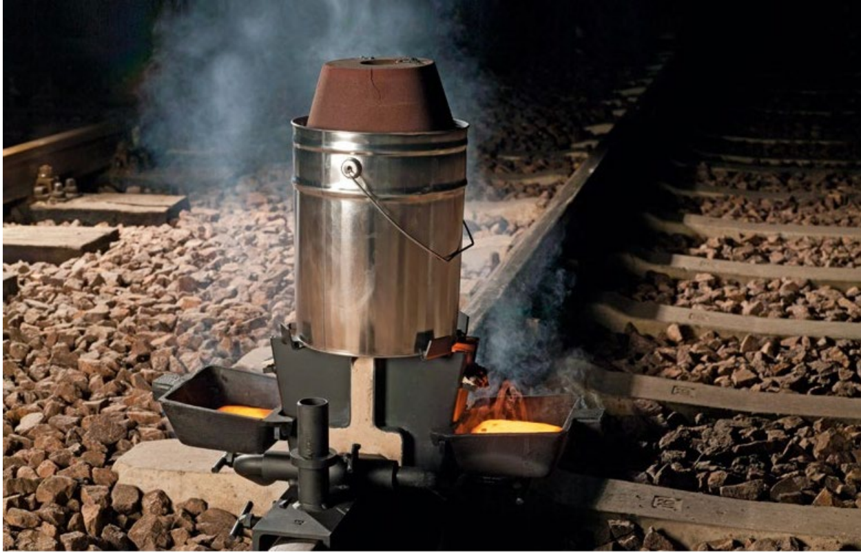
Figure 3. Thermite Field Weld Process (Source: mechanicalportal.com)
