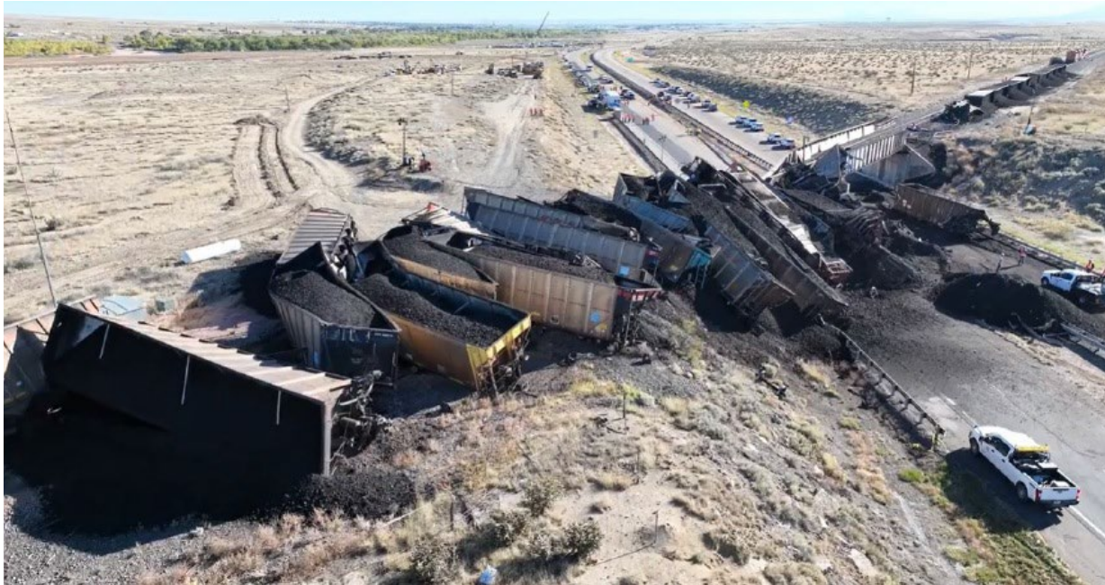
Figure 1. Aerial photo of the point of collision site. (source: BNSF Drone footage)
