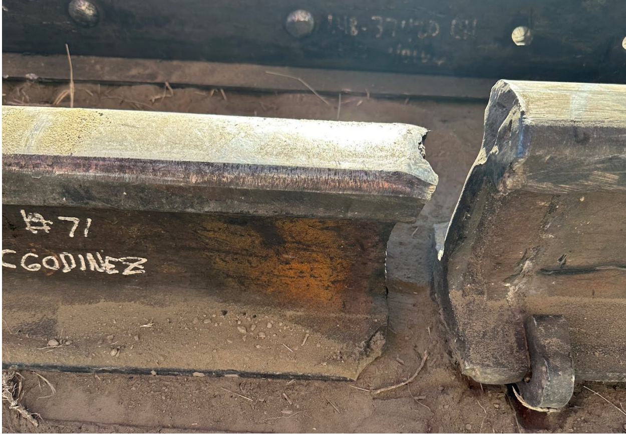
Figure 2. Thermite Field Weld #71 MP 109.656 made on 5-29-2023 (Source: NTSB)
