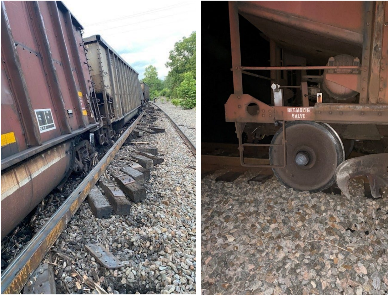
Figure. Derailed gondola cars ( left ) and a wheelset with a burned-off bearing ( right ). (Sources: NS ( left ); Federal Railroad Administration ( right ).)
