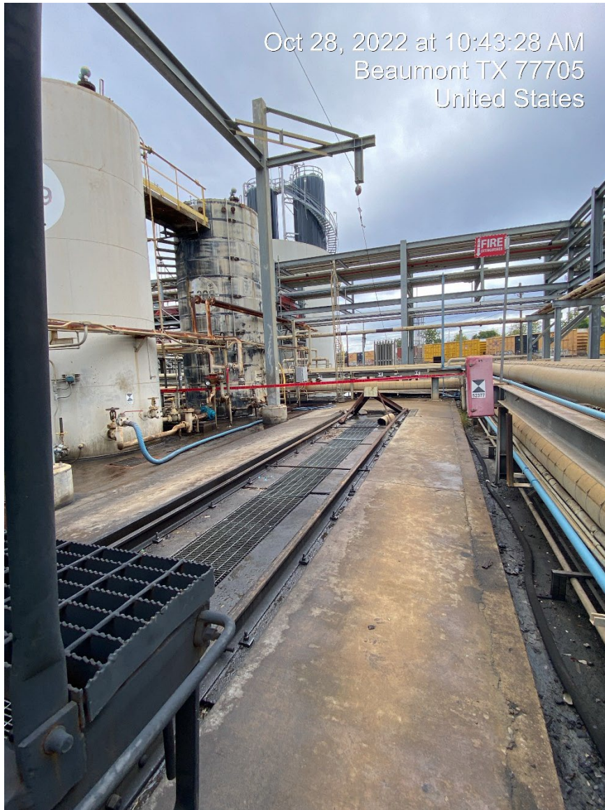
Figure 5: Distance from rear car to bumping post was measured at 35 feet.
