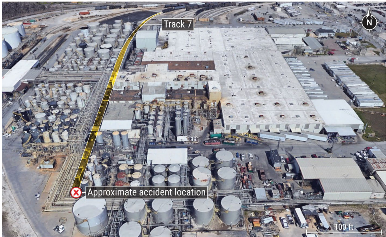
Figure 1: Satellite image of the accident location at the ExxonMobil lubricant plant. (Source: Google Earth Pro.)
