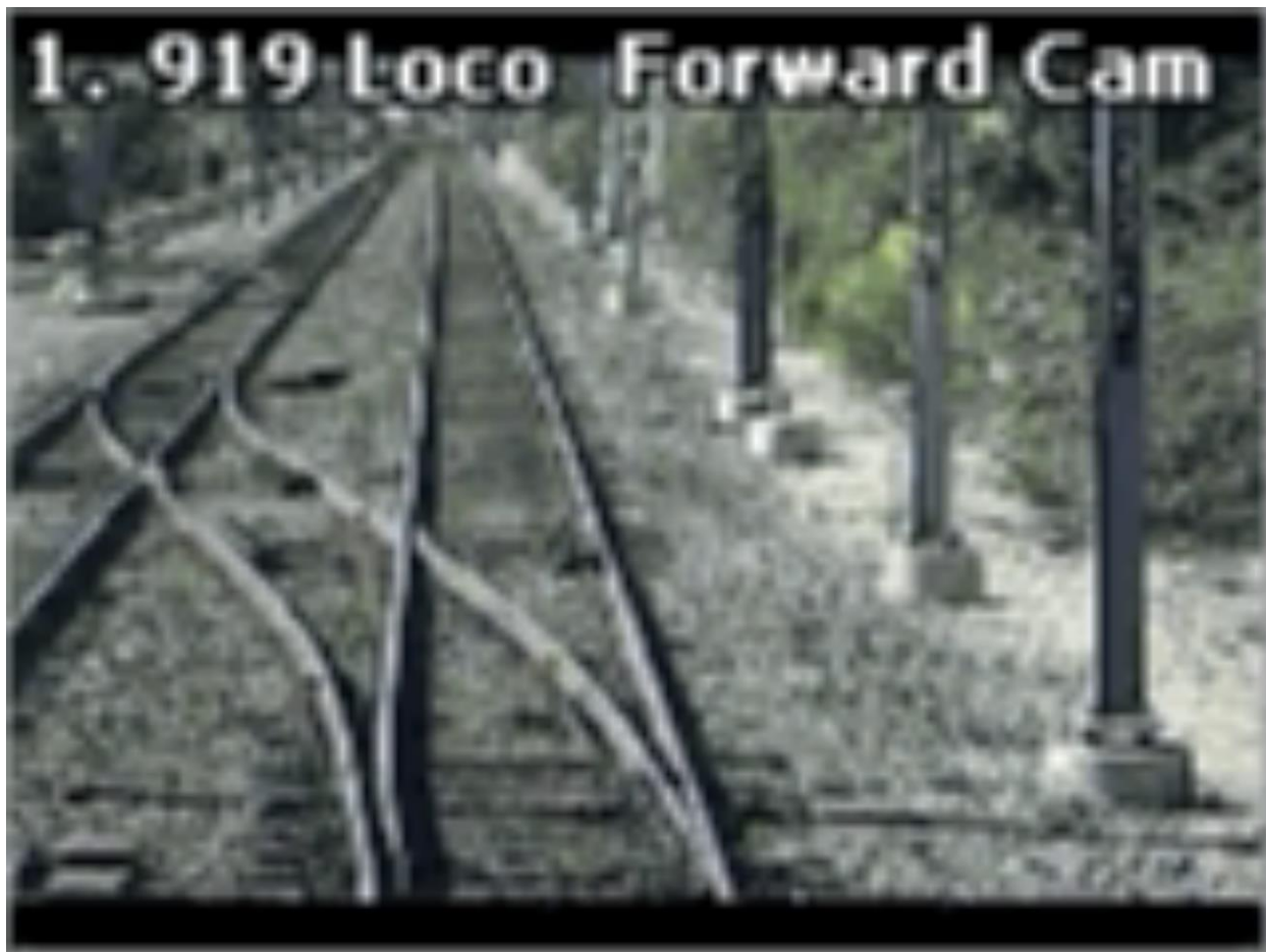
Figure 5. The view from the accident train approaching the crossover onto main track 1.
