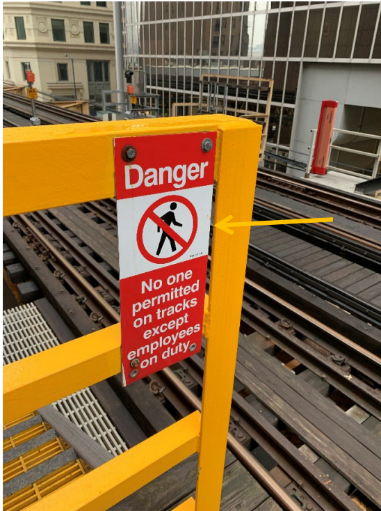
Figure 4: Photo showing no one permitted on tracks
