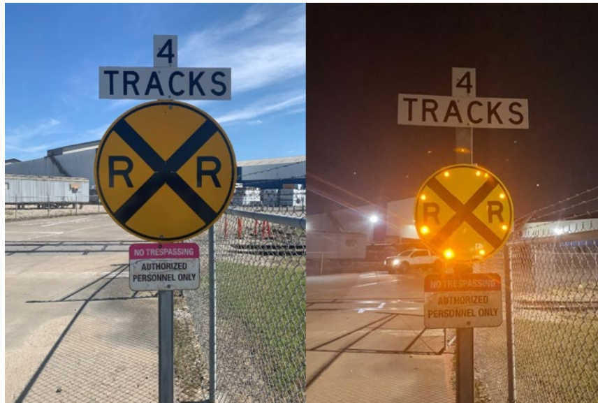
Figure 4: Looking in the direction of the movement of the combination vehicle, the two photos display the advance warning signage before and after the modification. The photo on the left was taken October 29, 2021, during the on-scene portion of the investigation. The photo on the right was taken on December 2, 2021, after completion of the modification to the advance warning signage.
