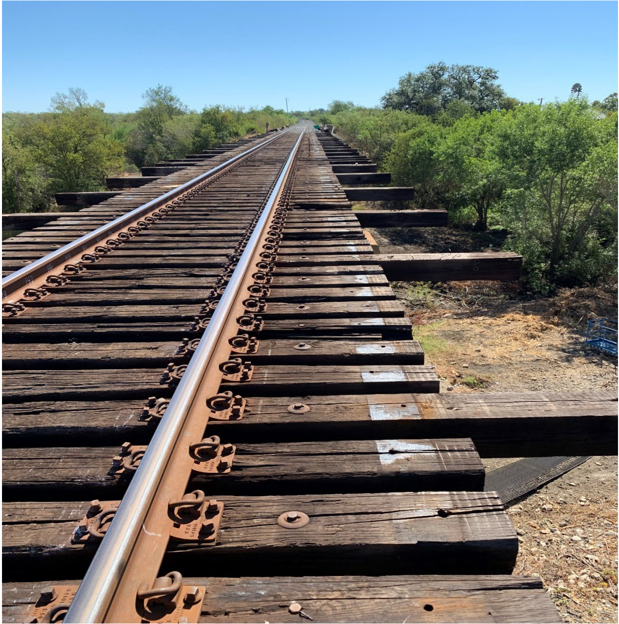
Figure 1- photo of Chacon Creek Bridge
