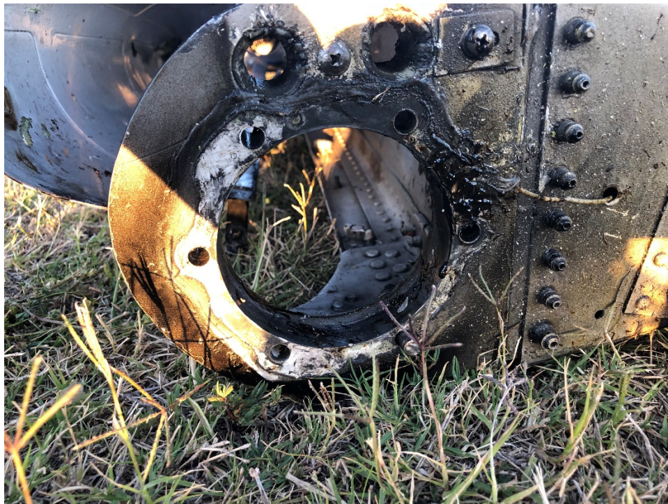
Figure 15: 90-Degree Gearbox Attachment Point on the Vertical Stabilizer
