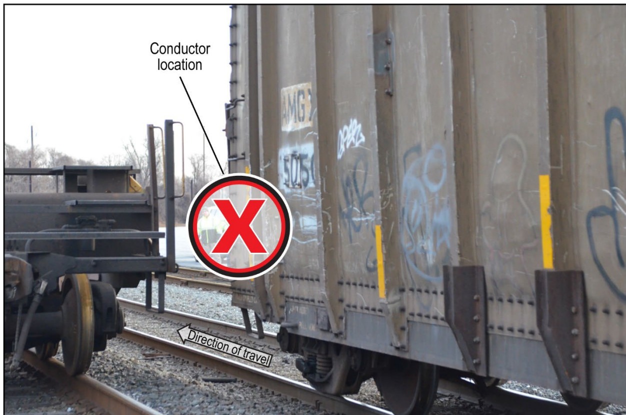
Figure 1. Accident railcar with the stationary railcar on adjacent track. (Photo courtesy of the Federal Railroad Administration (FRA).)
