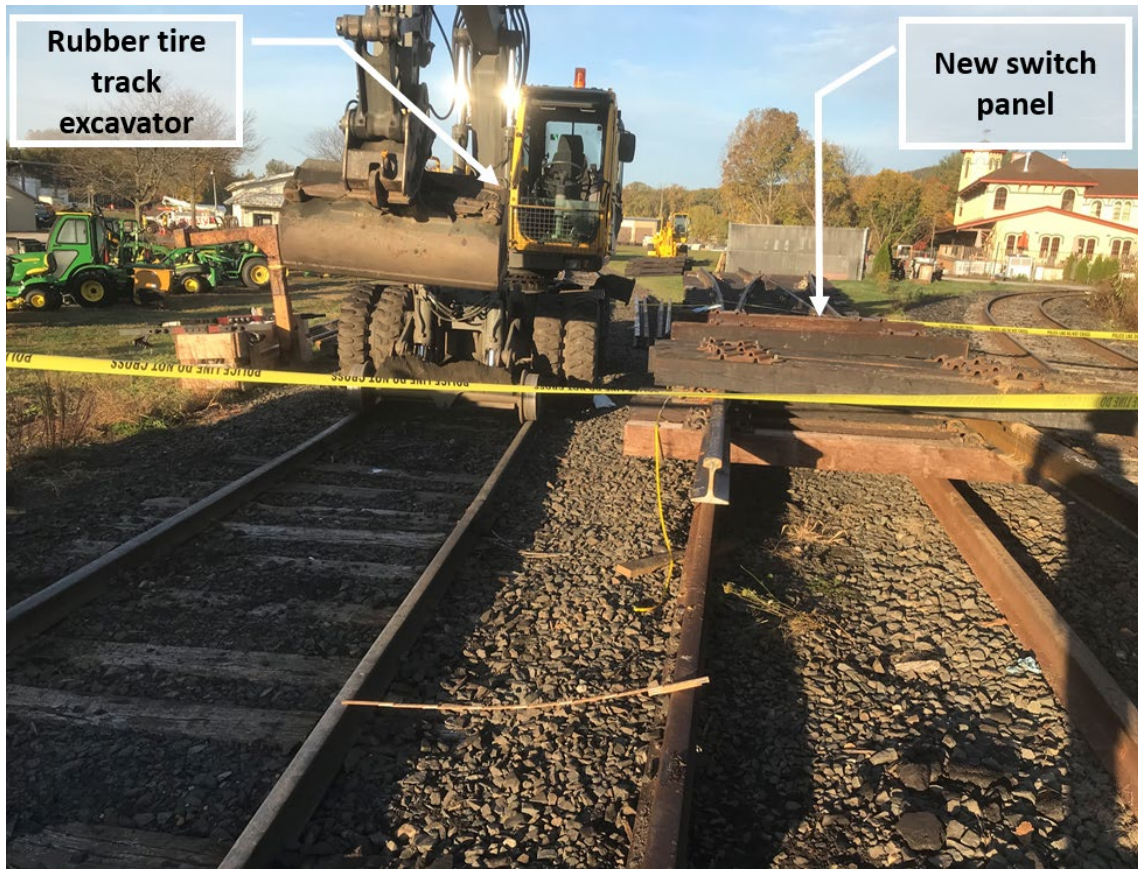
Figure 1. Location of the accident showing the excavator.
