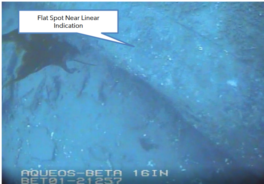
Figure 12. San Pedro Bay Pipeline linear indication with a Flat Spot in situ. Concrete rubble can be seen adjacent to the pipeline. Photograph by Beta Offshore, October 4, 2021.
