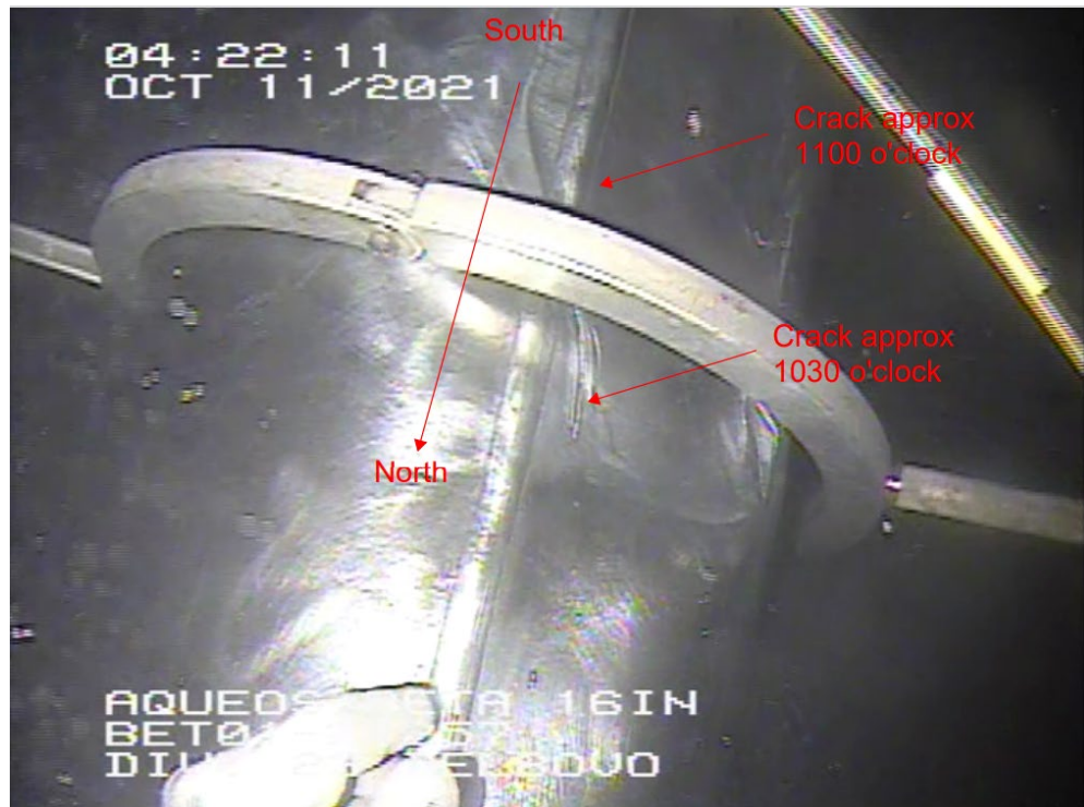
Figure 18. San Pedro Bay Pipeline Non-Destructive testing showing the crack location on the pipe. Photograph by Aqueos, October 11, 2021.
