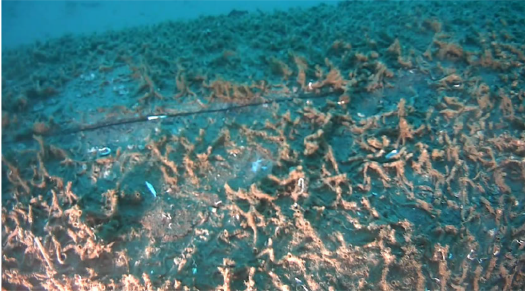
Figure 13. San Pedro Bay Pipeline linear indication at the release location with the coating in place. Marine growth is shown over the damaged portion of the pipeline. Photograph by Beta Offshore, October 4, 2021.
