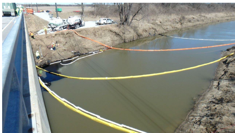
Figure 14. Oil recovery operations in Cahokia Creek upstream side of Wanda Road bridge, March 12, 2022, 12:12.
