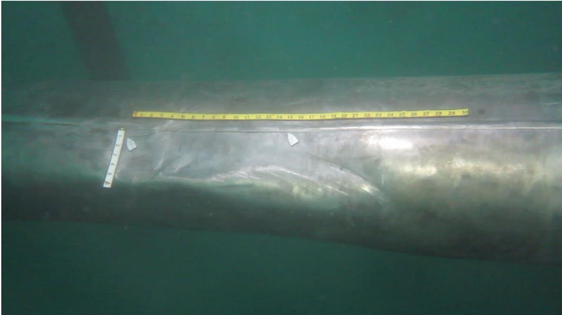
Figure 1: View of the pipe
