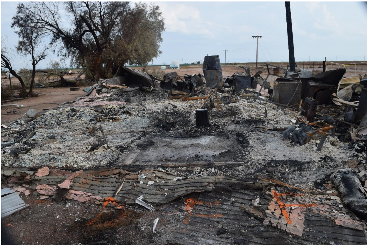
Figure 4: South wall looking north.
