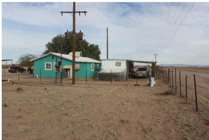
Figure 1: Residence from south (pre-fire)
