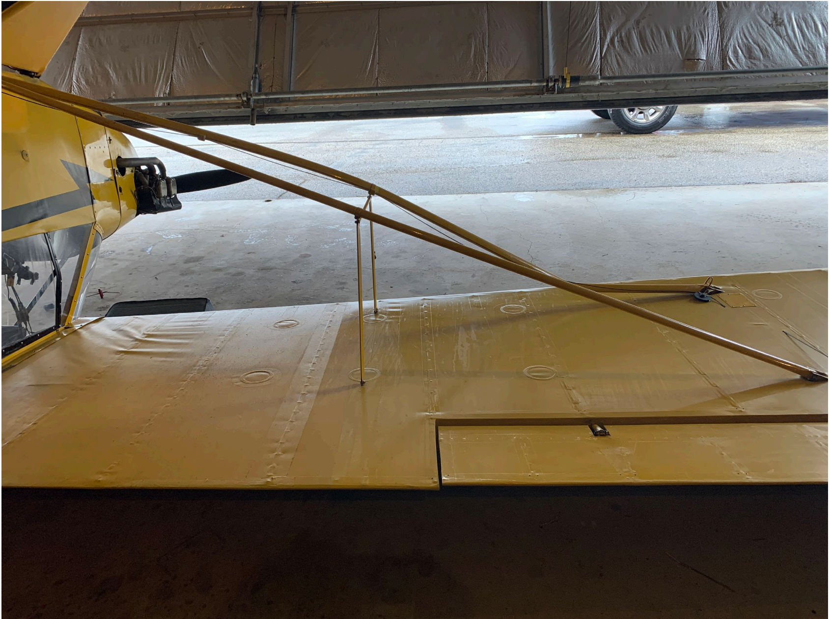
Photo 2 – Damaged Left Wing Strut, Courtesy of FAA
