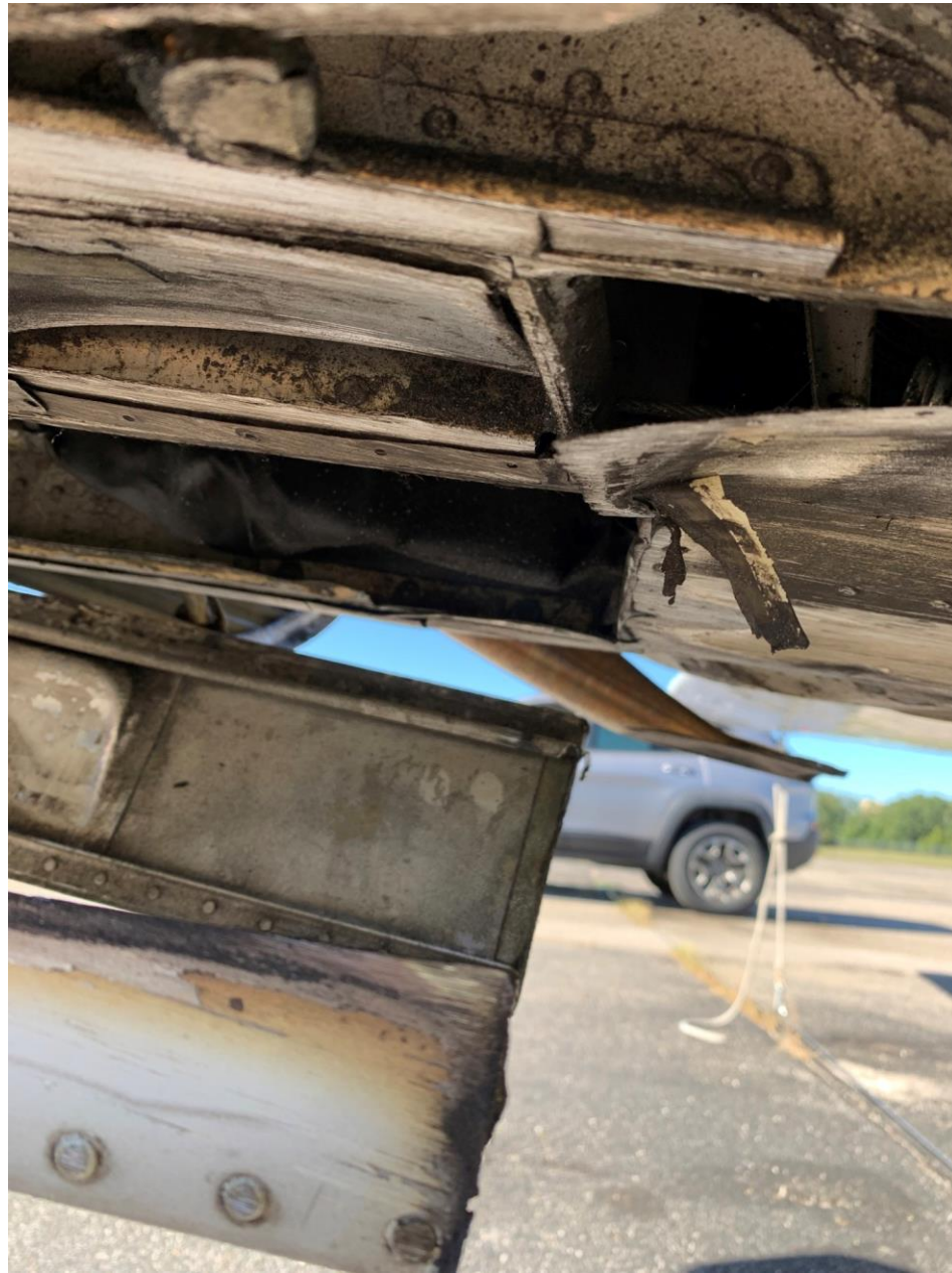
Photo 2 - Engine Keel Beam Damage (Courtesy of FAA)
