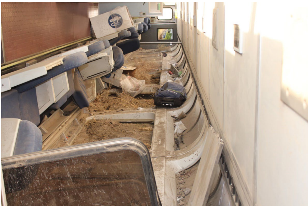
Figure 10 Photograph of the interior of the Lounge Car, ATK 33049, looking forward from the trailing end. The ground outside of the car is visible through the spaces created by the missing windows. (Source: NTSB)
