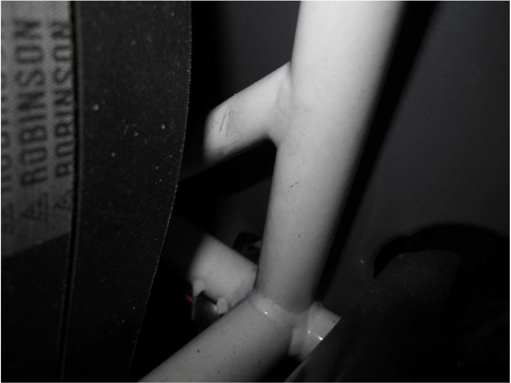
Photo 5 – Sheave Impact Mark
