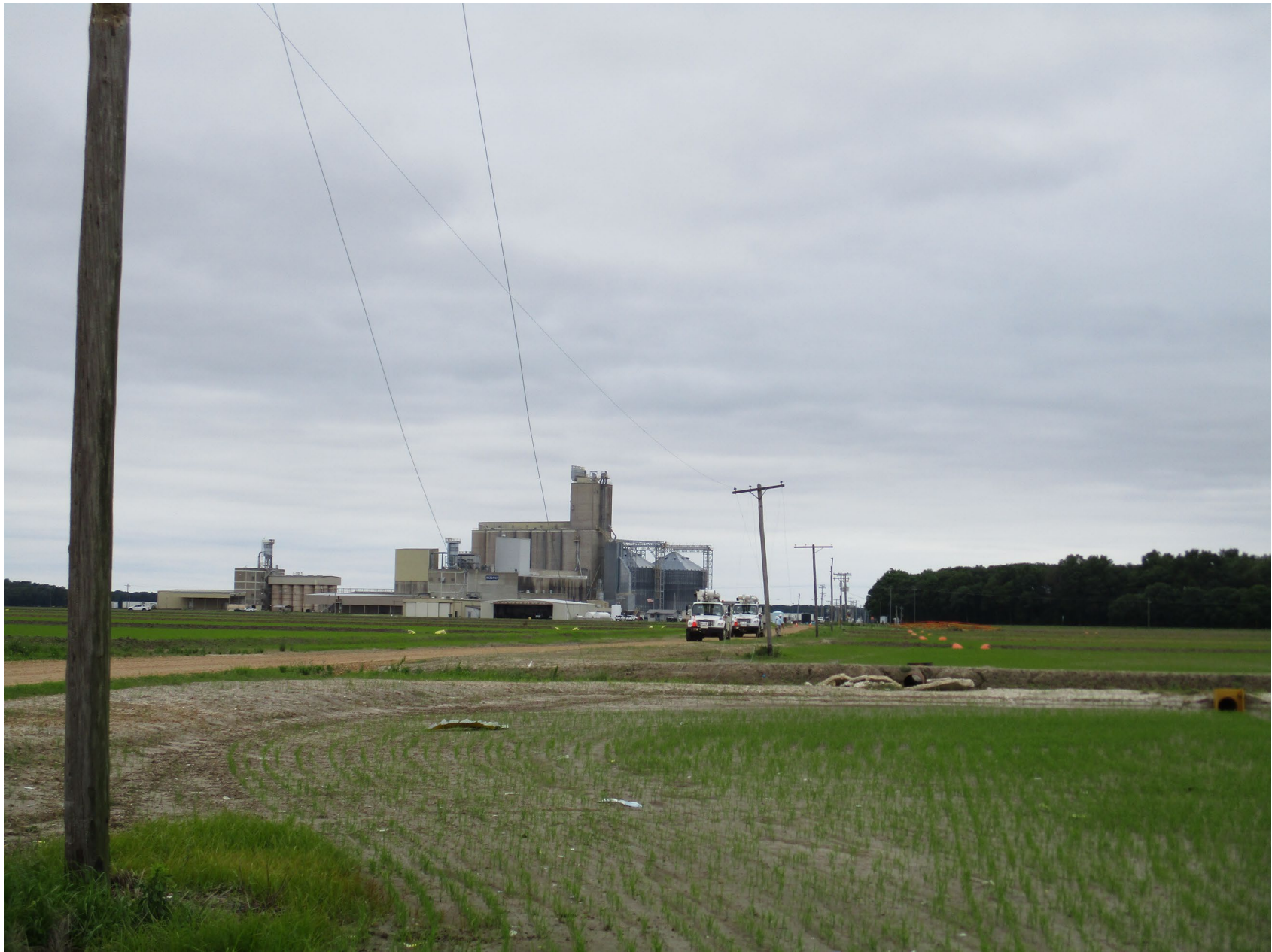
Photo 1 – Second Telephone Pole Impacted - Courtesy of FAA (Federal Aviation Administration)
