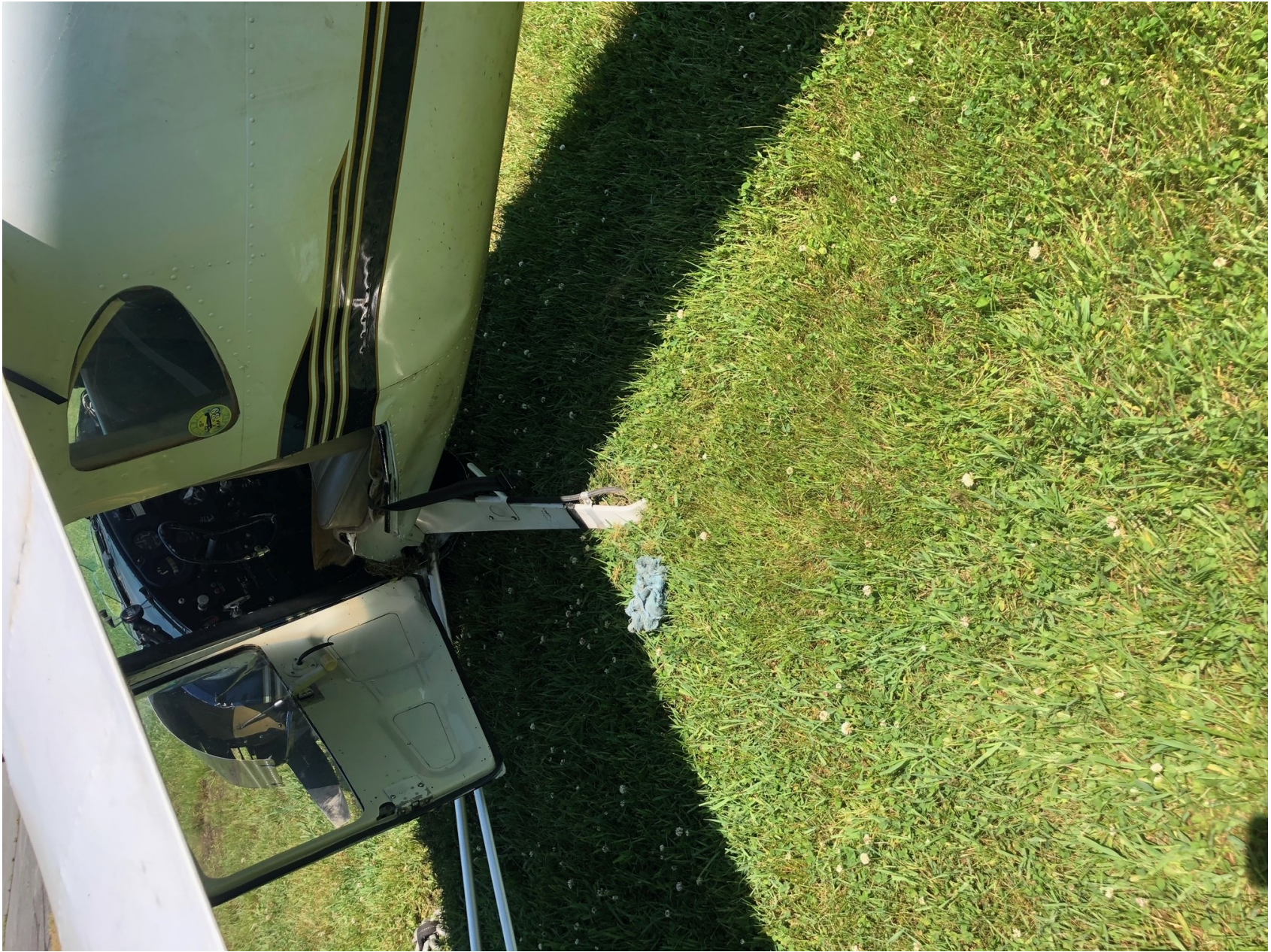
Photo 2 – View of left side of the fuselage showing buckling aft of door. (FAA Photo)
