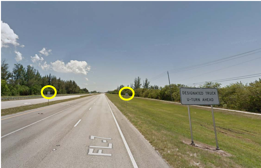
Photo #2 Google Street View image of southbound US 441 approximately 1 mile north of crash intersection. The image shows the posted 55 miles per hour speed limit signs (circled in yellow) and the advisory warning signs of turning trucks. Image captured May 2017.
