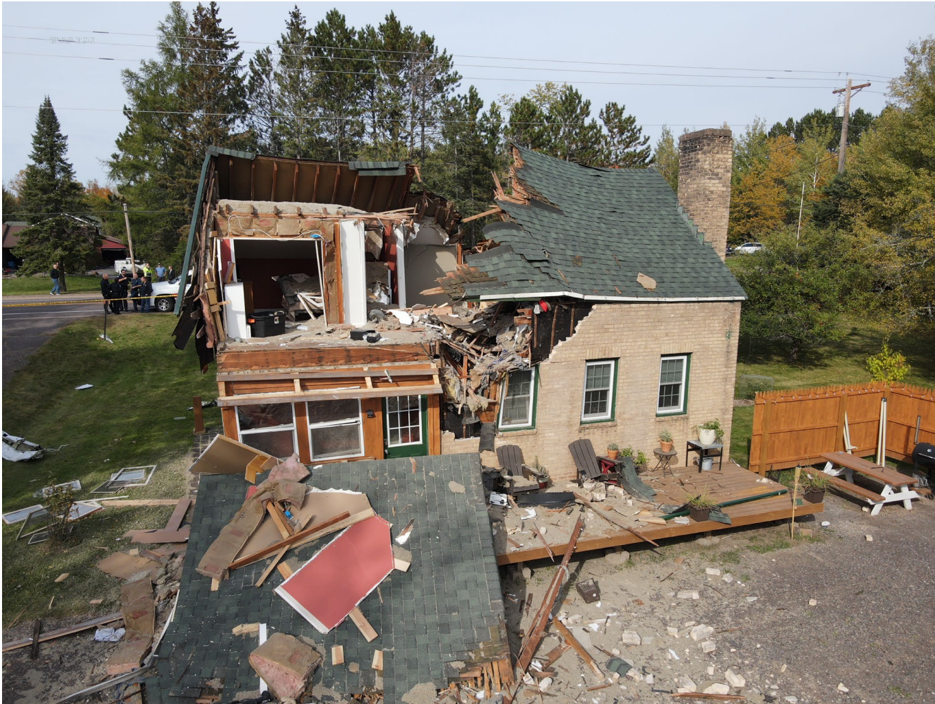
Photograph 2 - UAV aerial view of backside of house. (Courtesy of Hermantown PD)
