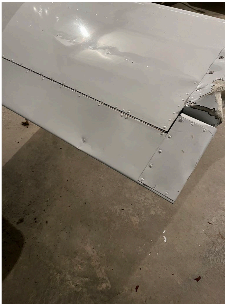
Photograph 3 - Right Elevator Damage (Courtesy of FAA)
