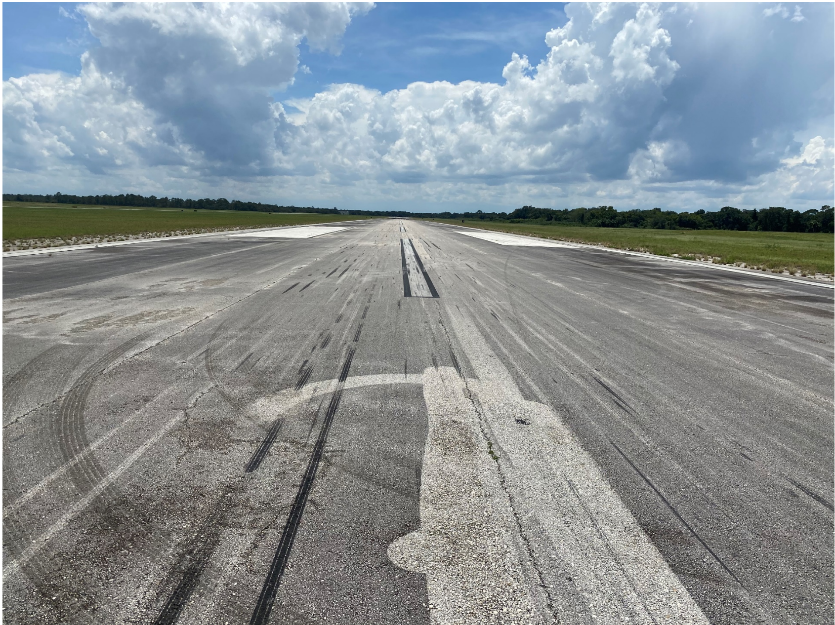
Photo 5 – View of Runway Skid Marks (Photo Courtesy of Space Coast Regional Airport Manager)
