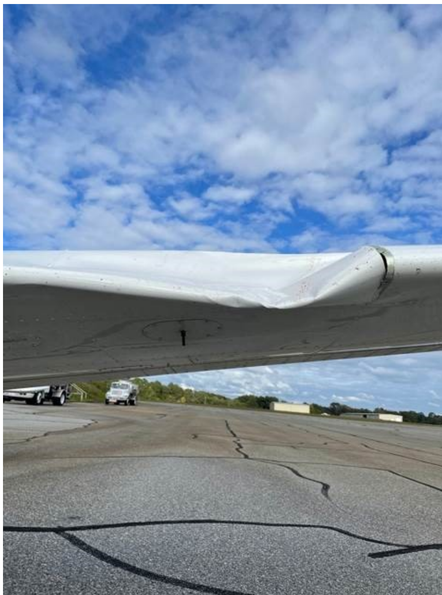
Photo 2 – Front view of left wind damage. (Courtesy of Operator)
