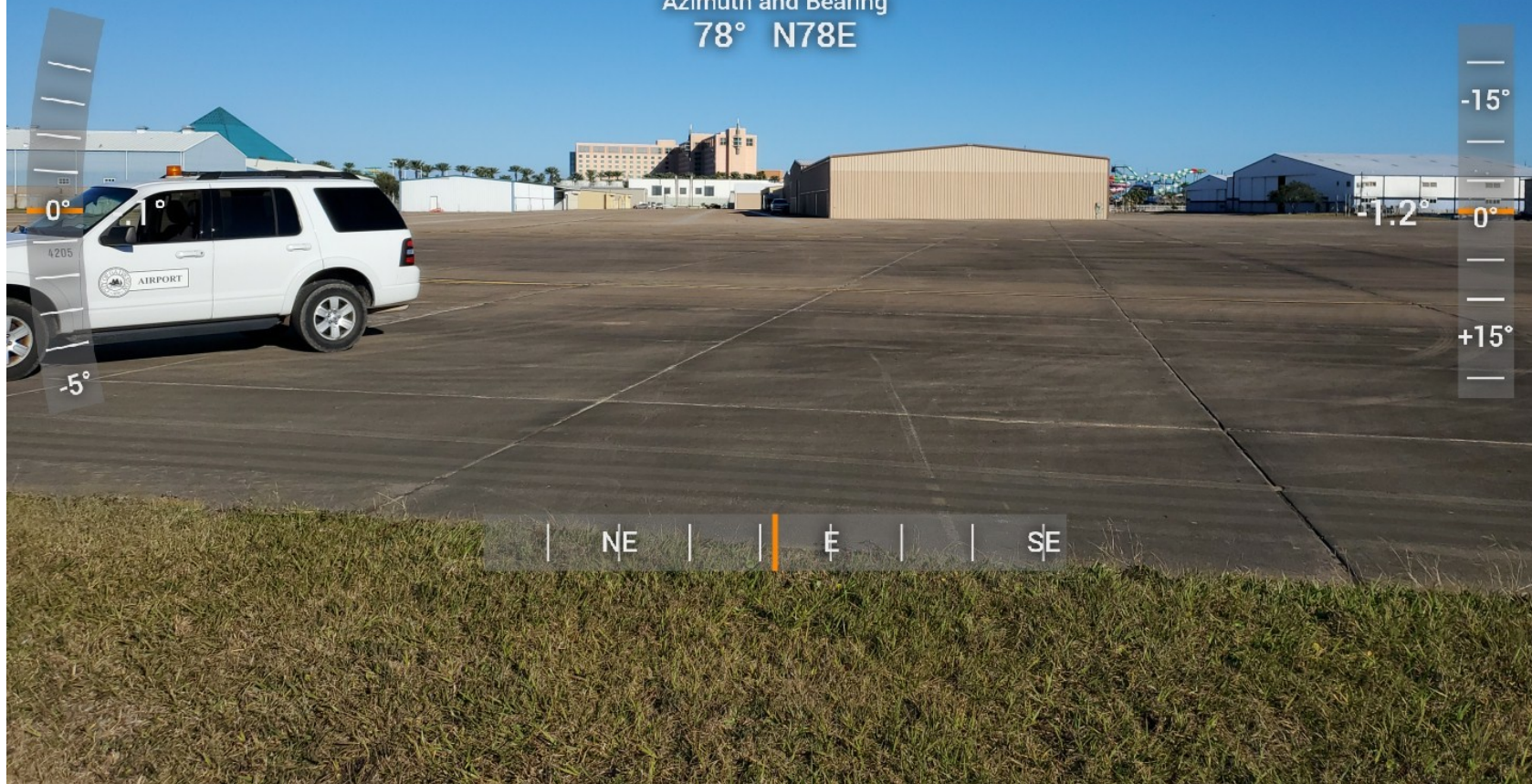
Photo 5 – Departure Ramp East View (FAA Photo)
