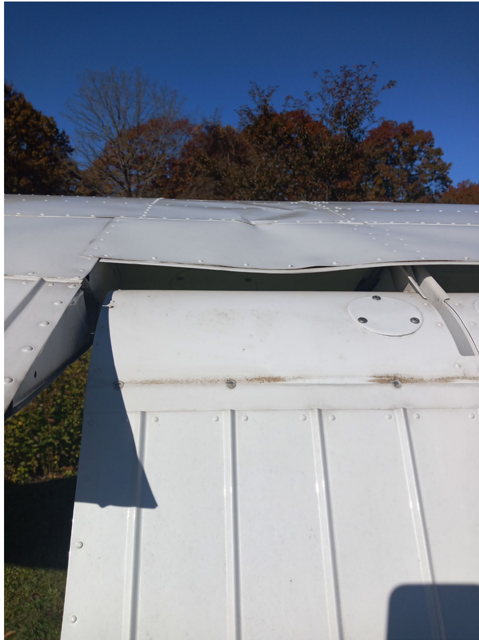
Photo 2 – View of left wing showing structural damage
