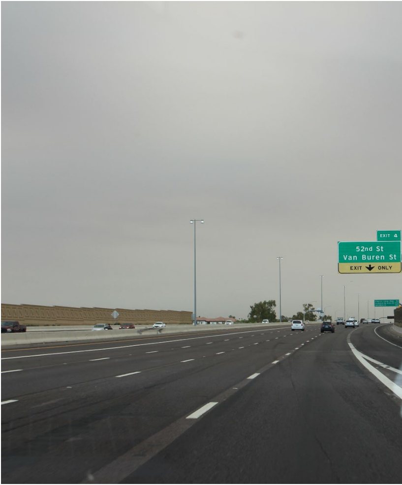
Highway Photo 5 – View of exit 4 ramp on eastbound SR Loop 202.
