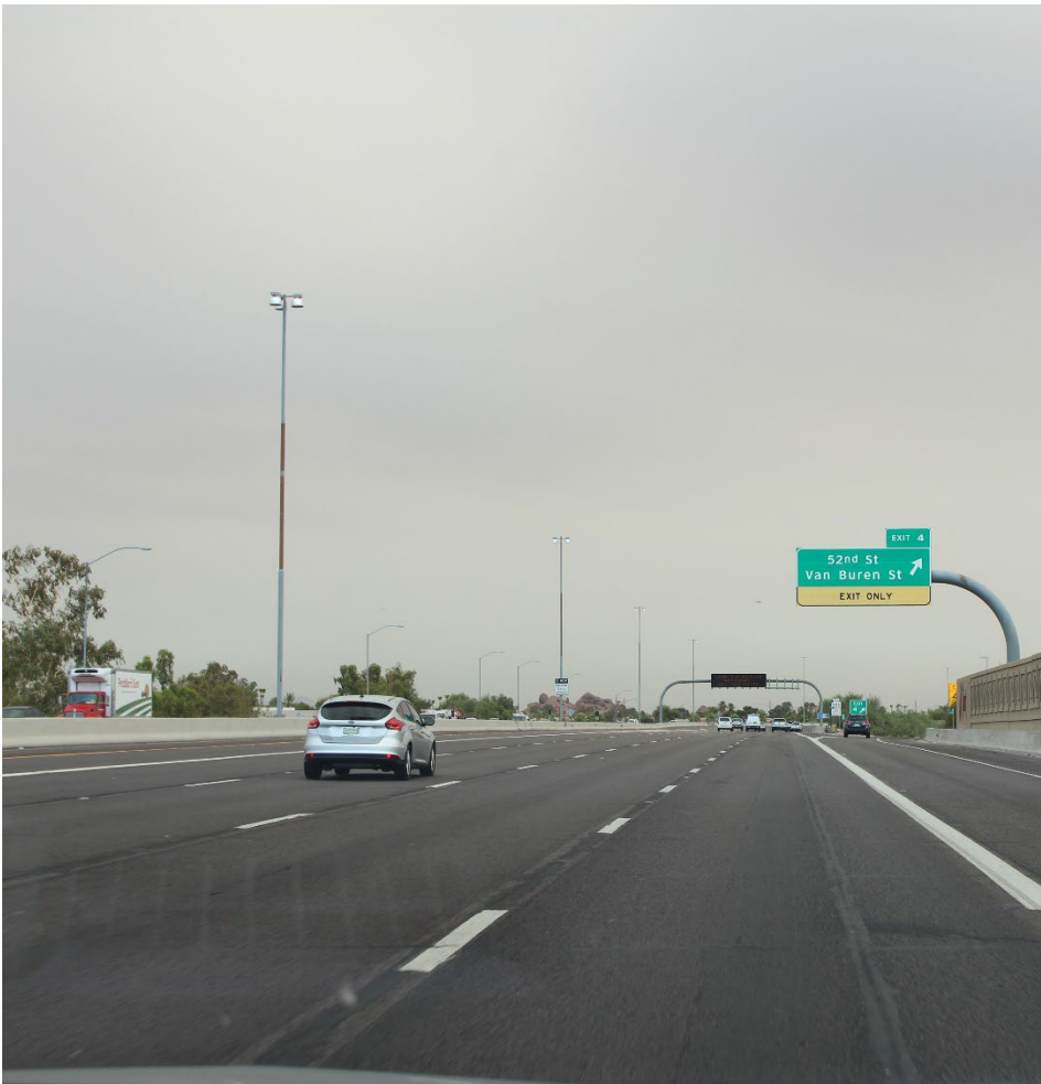
Highway Photo 7 – View of the exit 4 sign on SR Loop 202 eastbound with the crash location in the background near the second overhead DMS.
