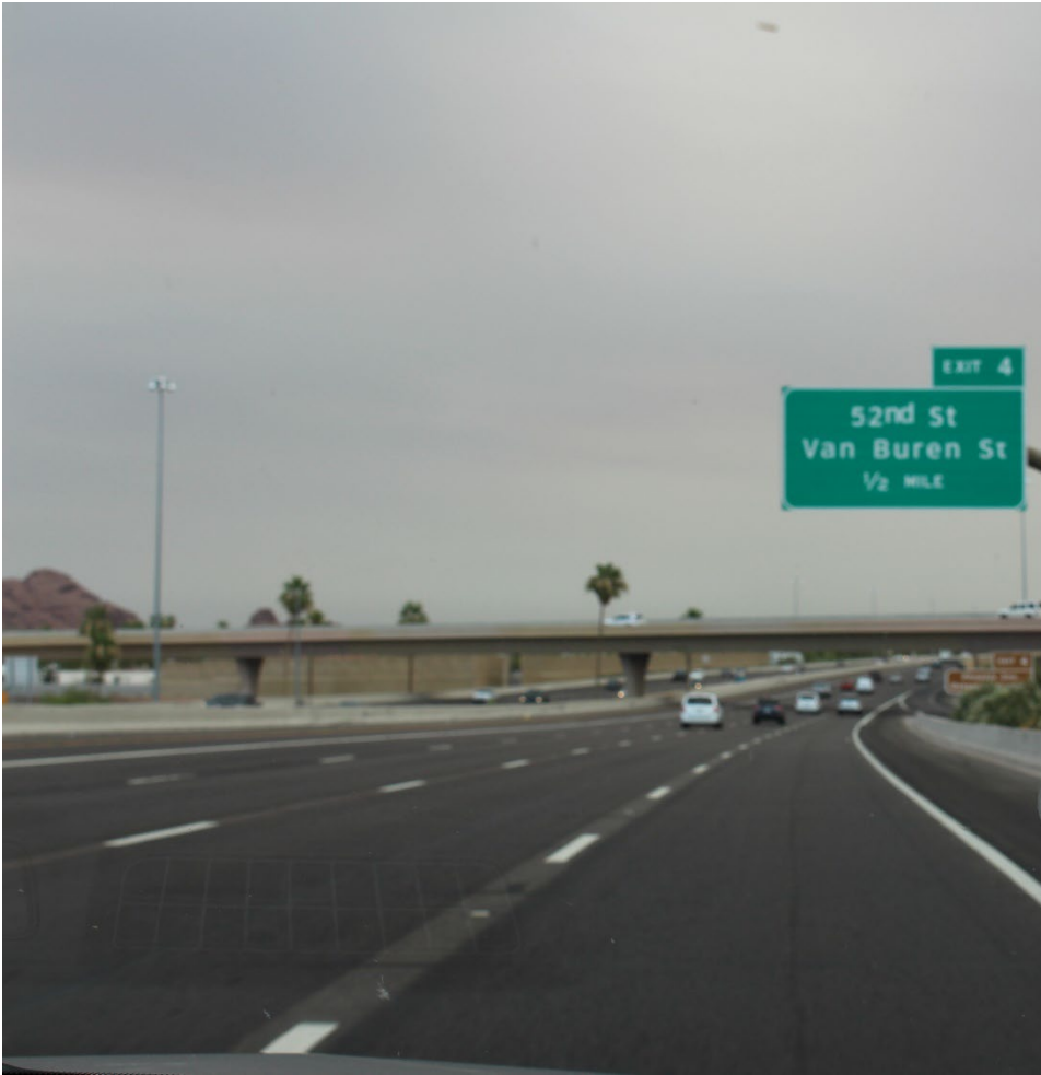
Highway Photo 4 – View of advance exit 4 sign on SR Loop 202 eastbound, approximately ½ mile from the exit ramp.
