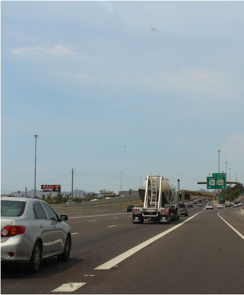
Highway Photo 1- This photo shows SR Loop 202 exit from I-10.
