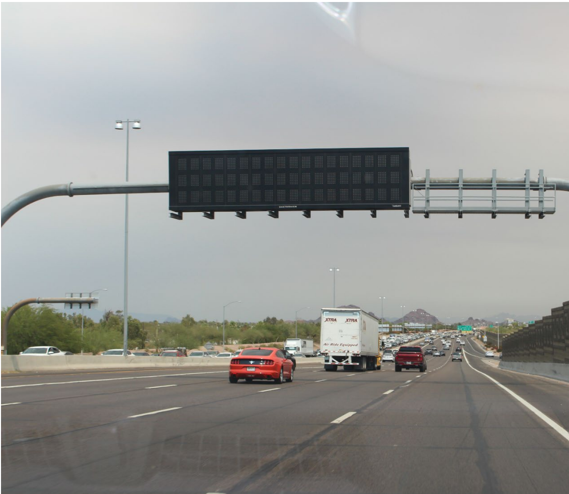
Highway Photo 3 – Close-up view of DMS at mile marker 1.75 on eastbound Loop 202.
