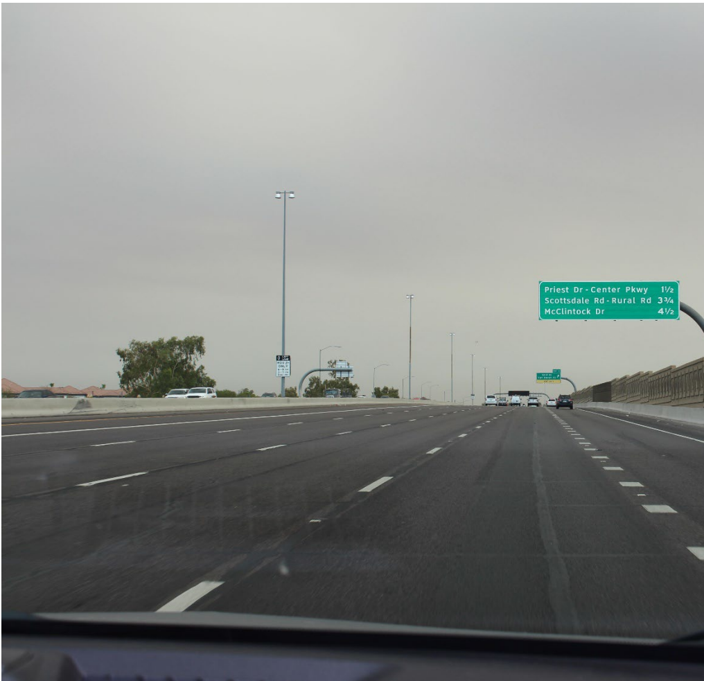
Highway Photo 6 –View of advance exit sign for Priest drive exit where the Traffic Incident Management area was located closing the eastbound Loop 202 lanes.
