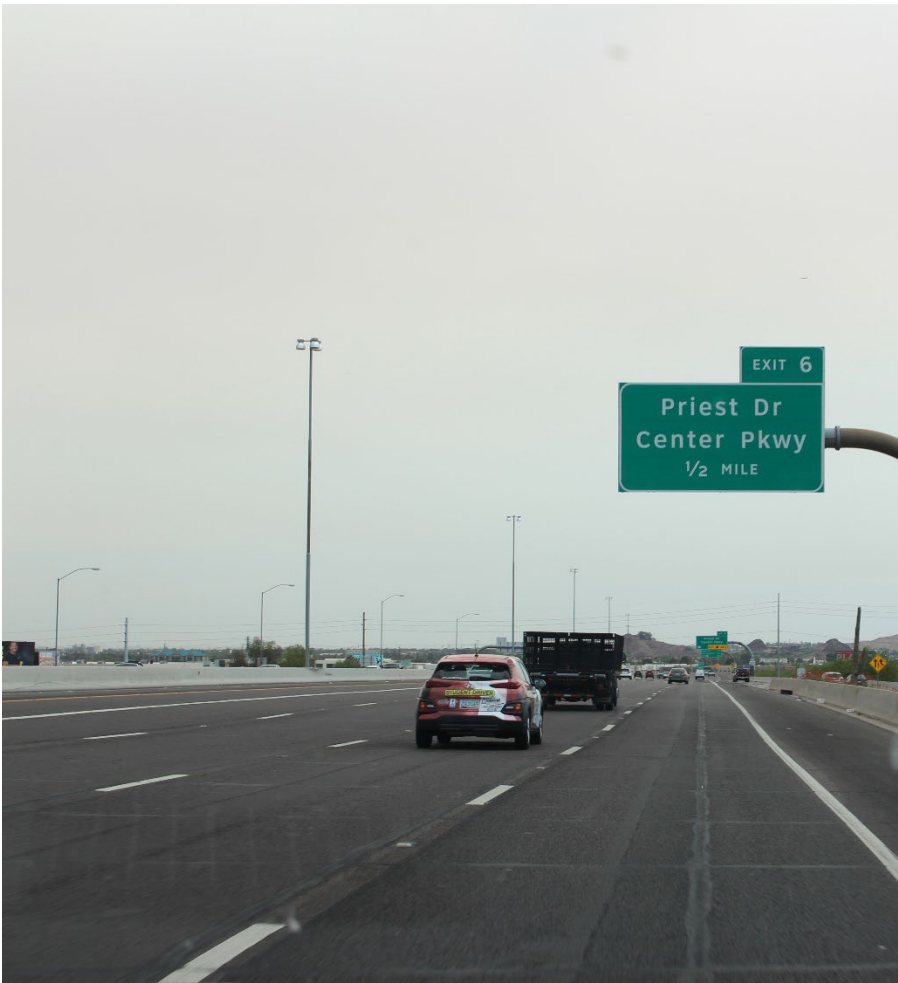
Highway Photo 9 – View of advance exit sign for exit 6 Priest Dr., approximately ½ mile from the beginning of the exit ramp on eastbound Loop 202.
