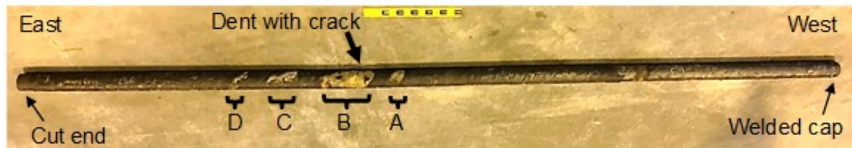
Figure 10. Natural gas main recovered near 3539 Durango Drive sewer lateral crossing.
