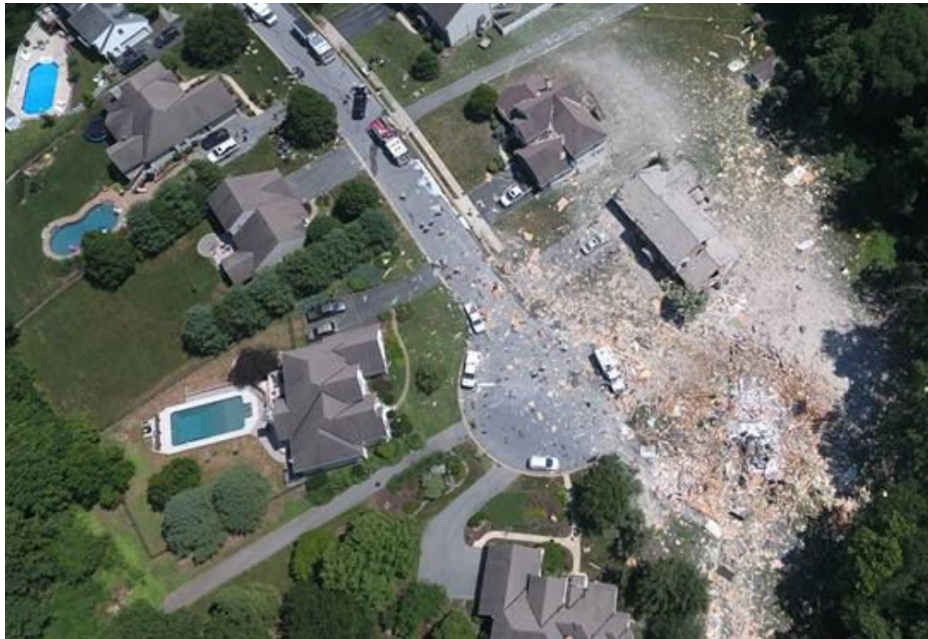
Figure 1. Debris field at cul-de-sac area where explosion occurred.
