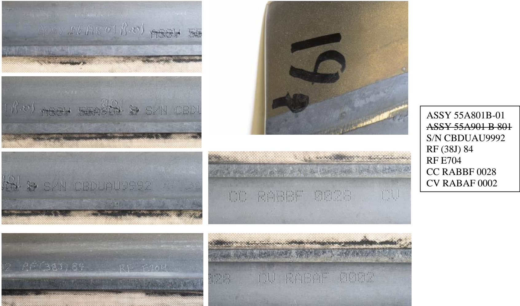
Figure 2: Images of the part markings observed on the root bottom of the fractured blade.
